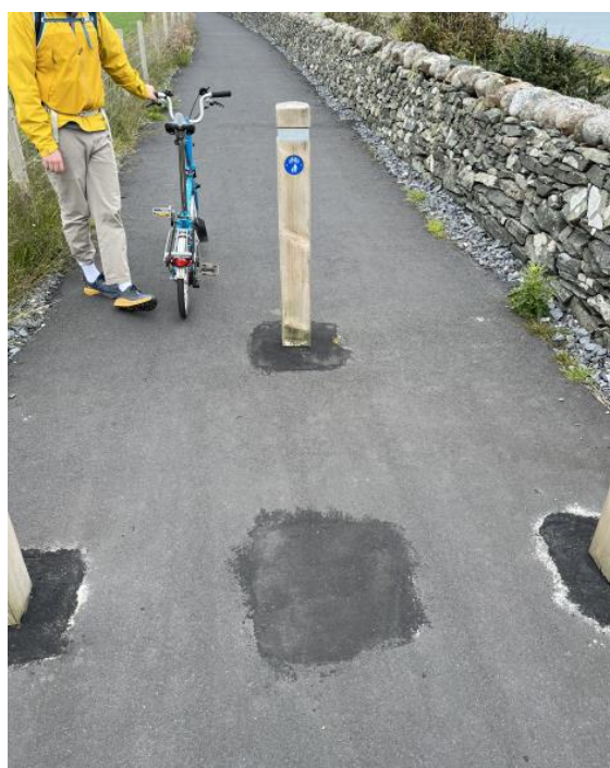
Re-positioned bollards at the entrance onto the Lochindaal Way
